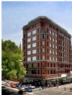
SYDNEY CENTRAL YHA (Heritage Department Store conversion)
