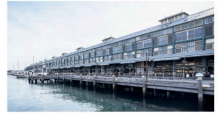
WOOLLOOMOOLOO WHARF (OVOLO) HOTEL (Heritage Wharf Woolstore Conversion)
